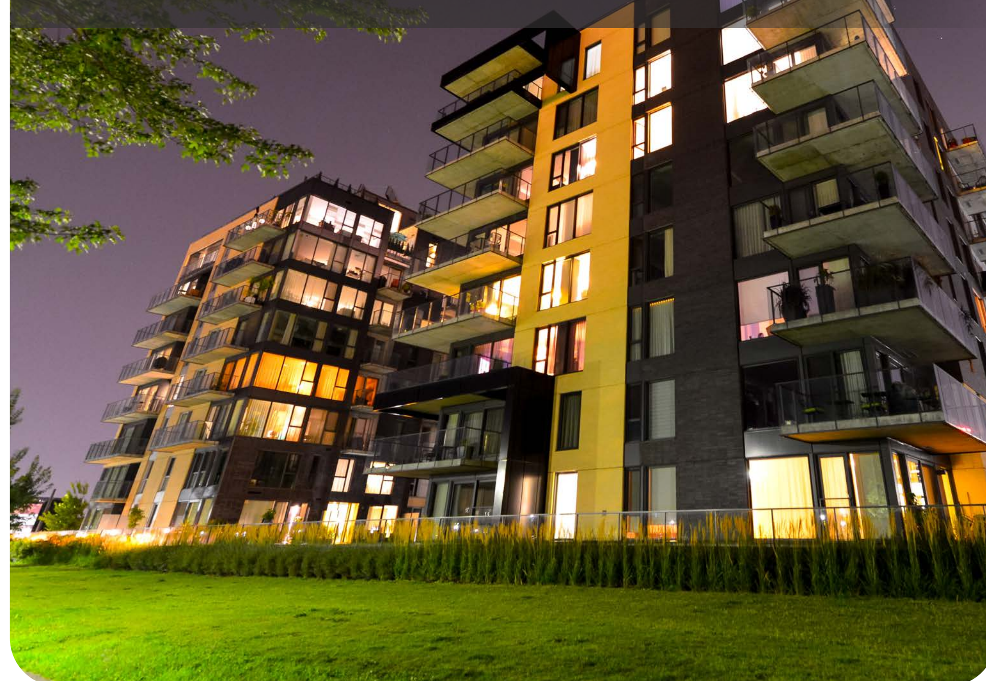
LES BASSINS, MONTREAL, QUEBEC
