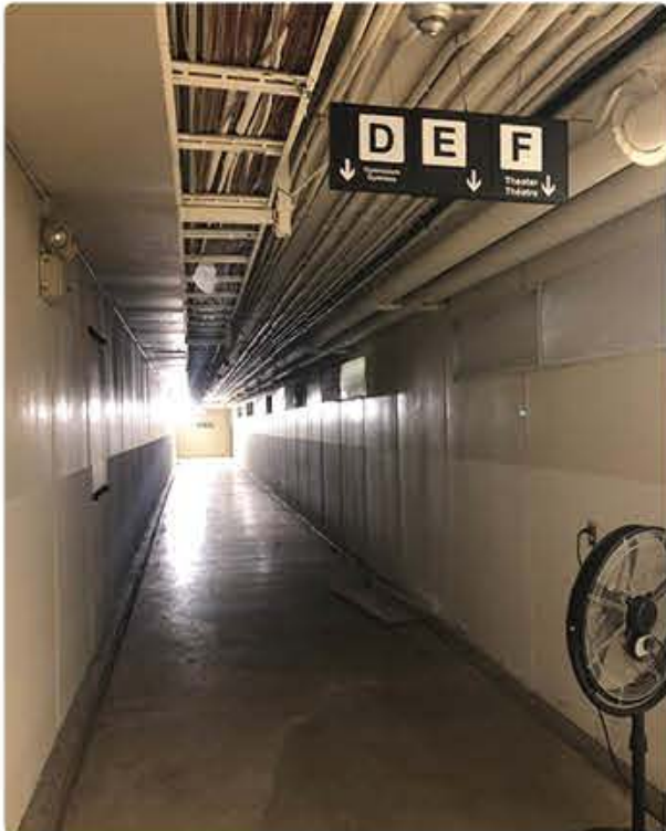
Underground Corridor / Corridor souterrain [ERA, 2021]
